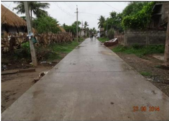
Figure 5: Road at Dindi, Andhra Pradesh
