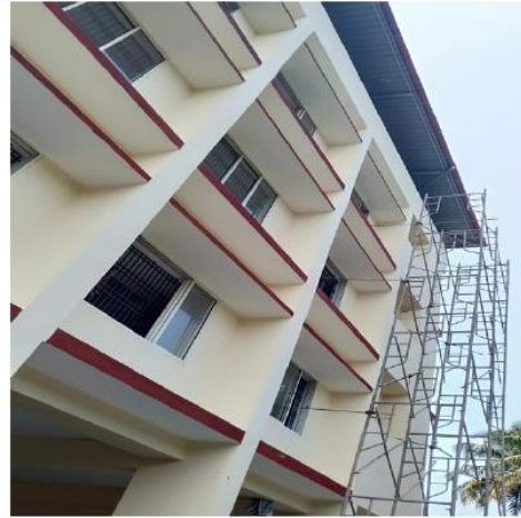
Figure 8: MPCS at Hosebette, Karnataka
