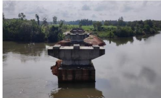
Figure 6: Bridge work under progress at Udupi, Karnataka
