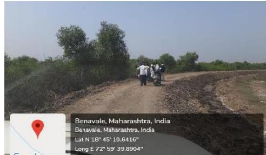
Figure 4: SE work under progress at Benavale, Maharashtra
