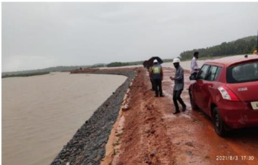
Figure 5: SE work under progress at Manikatta, Karnataka
