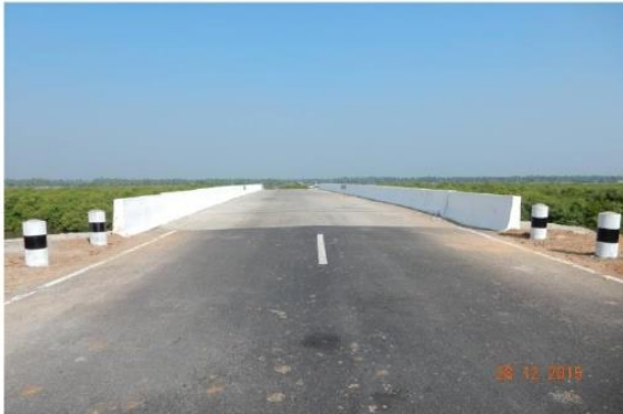
Figure 1: Bridge at Narayanapuram, Andhra Pradesh
