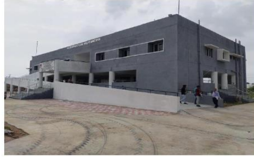
Figure 2: MPCPS at Maktupur, Gujarat
