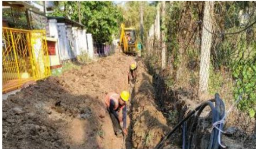
Figure 3: UGC work under progress at Alibag, Maharashtra
